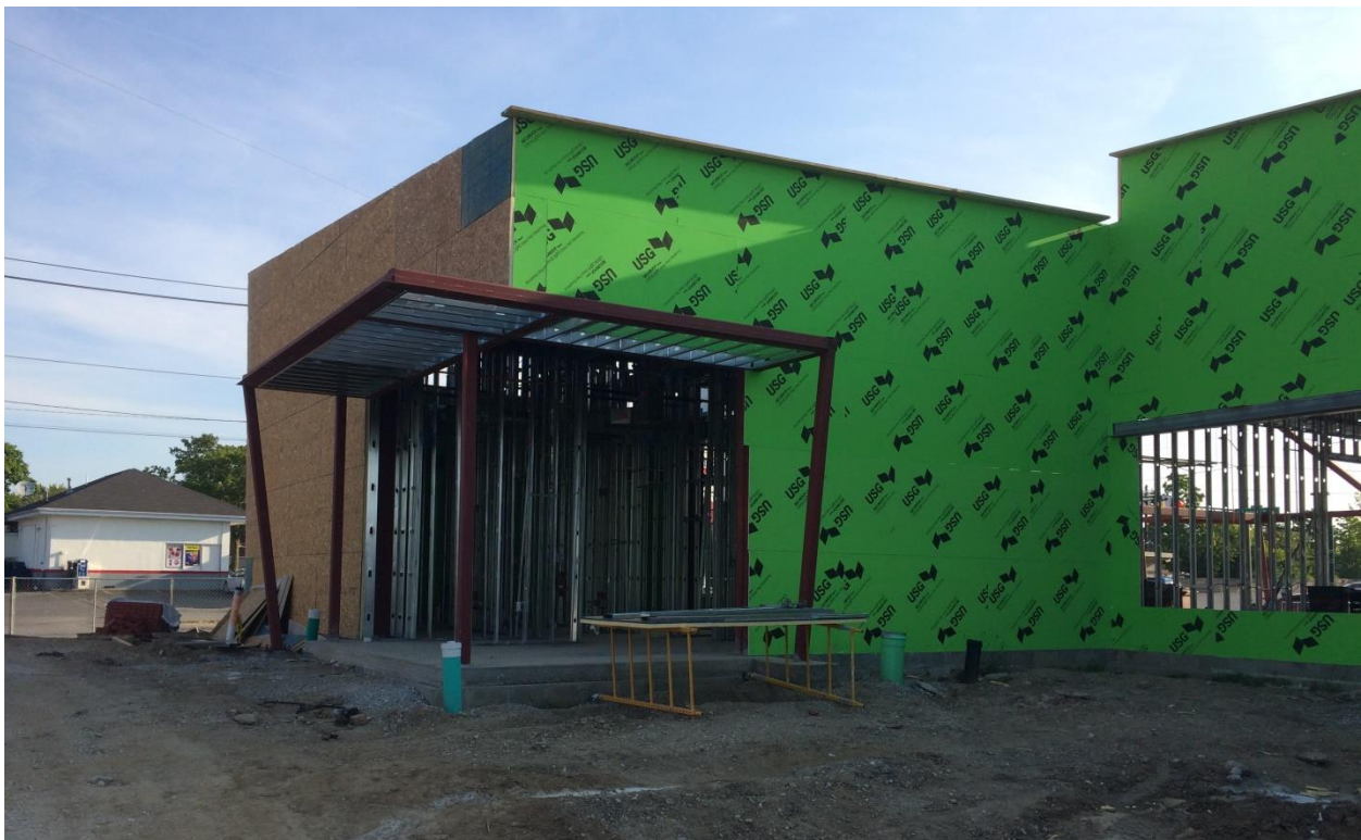
Project Site on September 9, 2019 Exterior view of the west entrance.
