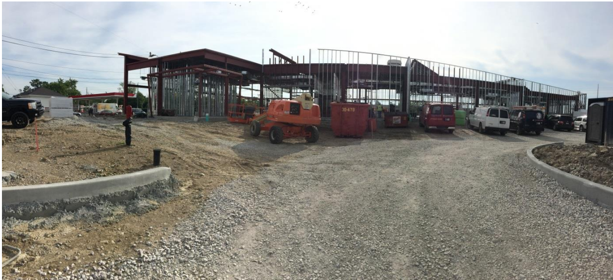
Project Site on August 9, 2019 Exterior panoramic view of the west side of the building.
