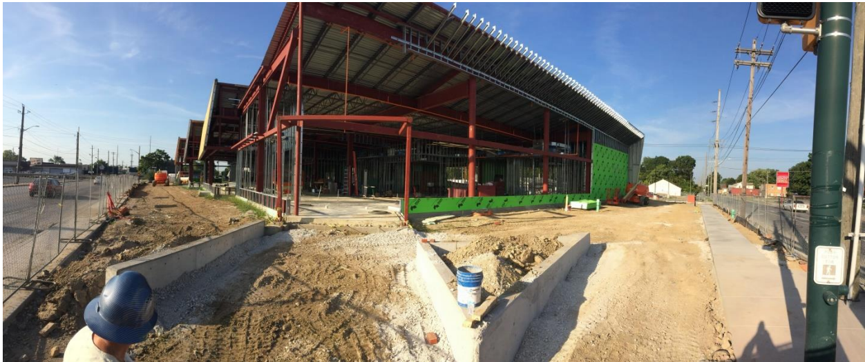
Project Site on September 9, 2019 Exterior panoramic view of the Sherman entrance.
